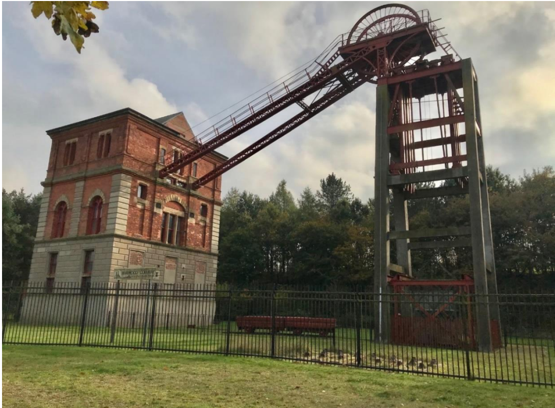
Photo 3: Winding Engine House – Grade II* Listed Building and Scheduled Monument
