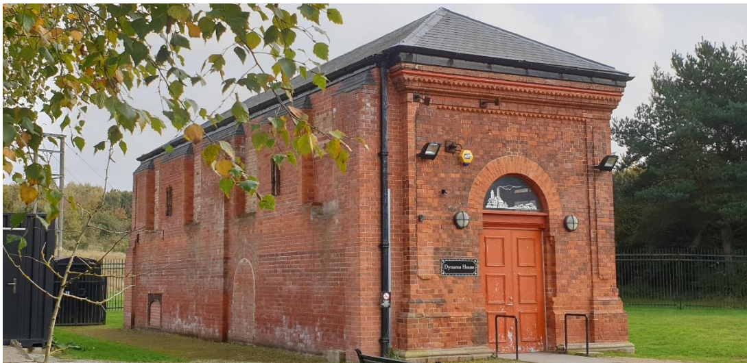
Photo 4: Dynamo House (former electricity substation)
