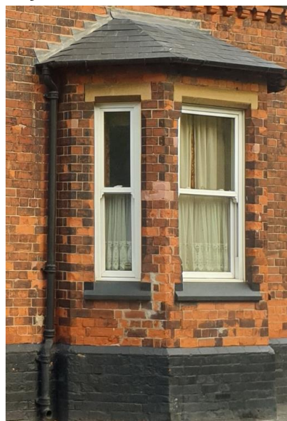
Photo 27: Brick wall in English Bond having alternating courses of headers and stretchers
