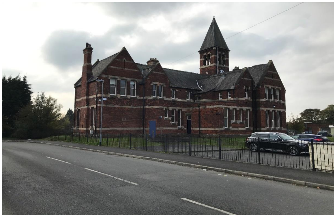
Photo 29: Former Bestwood Coal and Iron Company offices
