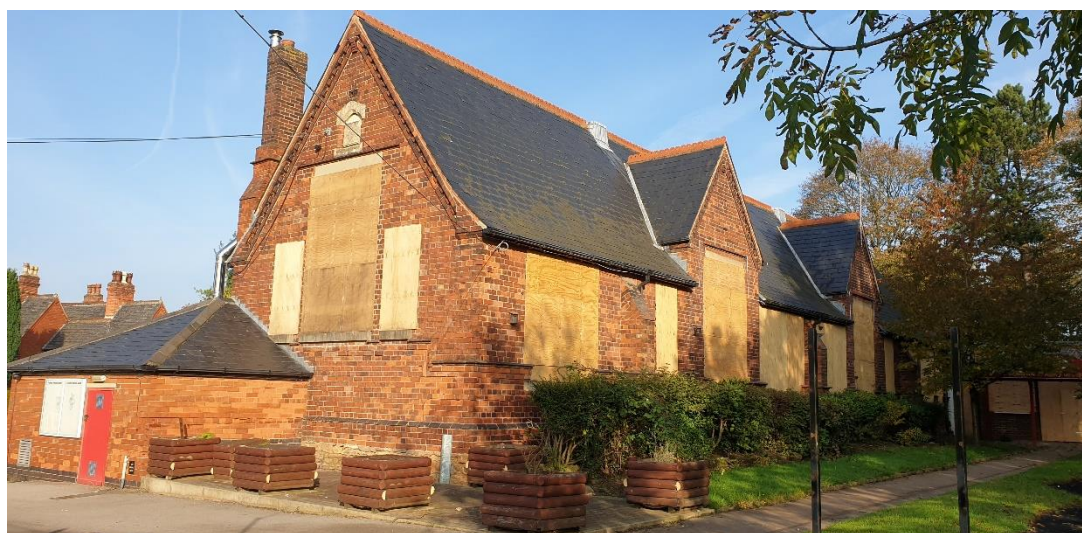
Photo 22: Former Hawthorne Primary School
