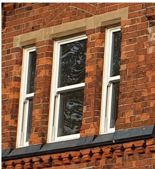
Photo 27: Brick wall in English Bond having alternating courses of headers and stretchers
